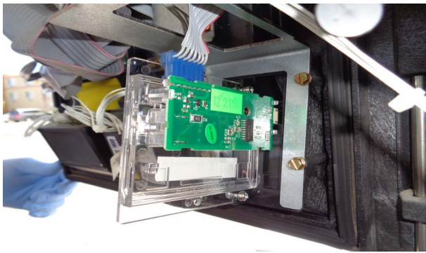
A skimmer installed inside an ATM. Photo courtesy of Henderson Police Department
